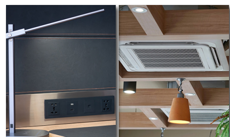
Office outlets Heating system
